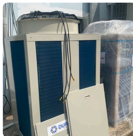
Outdoor unit maintenance at a factory
