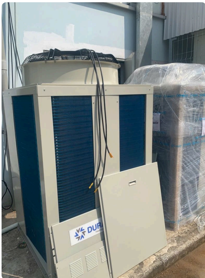
Opening the Durate AHU condensing unit before charging
