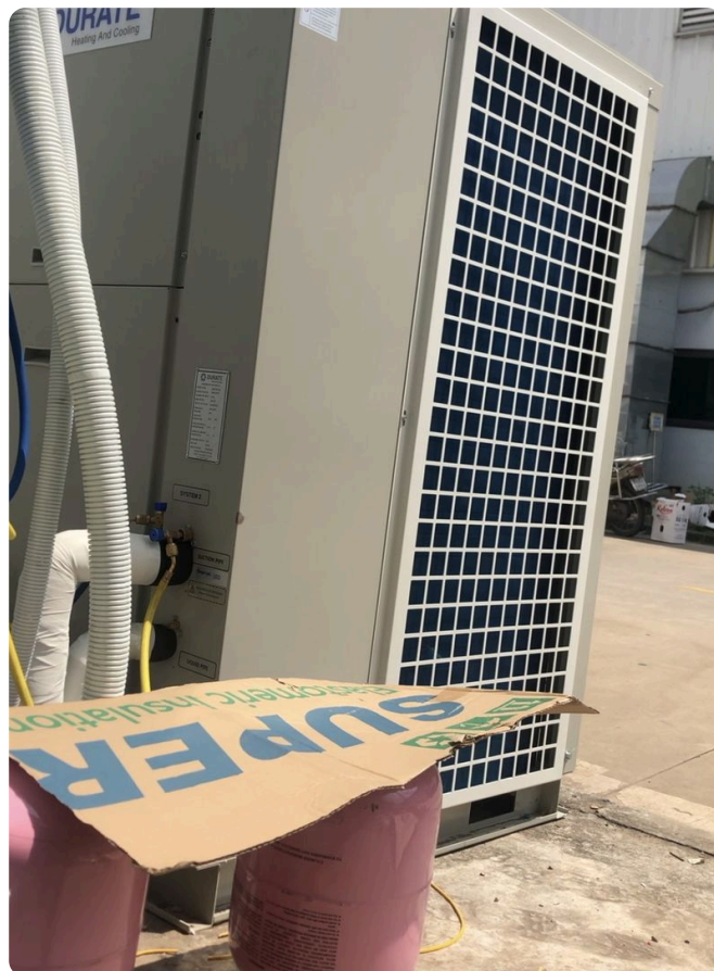
Charging R410A into the Durate AHU condensing unit
